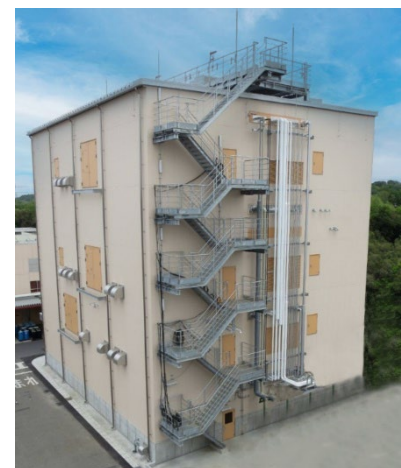
▲ Completed production facility (ADEKA CORP. Chiba Plant)
