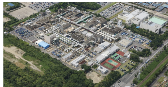
▲ Chiba Plant view
