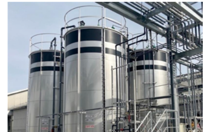
High-purity hydrogen peroxide for semiconductors (New plant construction)
