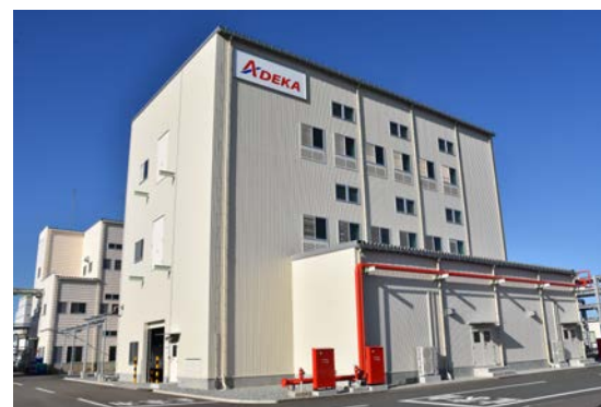
▲ Soma Plant: Facilities for lubricants
