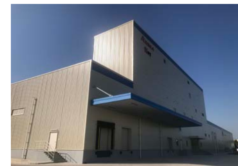
▲ New manufacturing building for manufacturing of processed foods [ADEKA FOODS (CHANGSHU) CO., LTD.]
