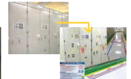
Displaying of wiring path and procedures on power receiver panels allowing anyone to restore power during blackouts
