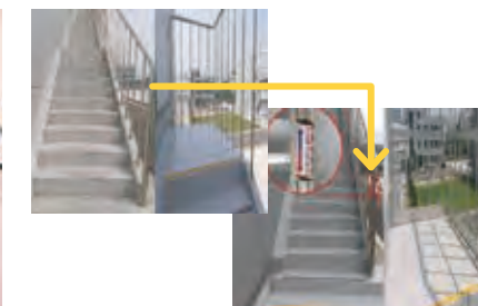
Stairs are given slip resistant surfaces to prevent slipping, and a fence is erected along the side to prevent secondary accidents
