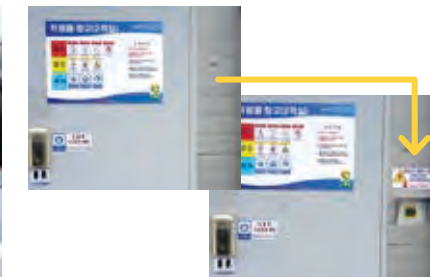
Installing a static electricity removal sheet in front of dangerous goods warehouses to eliminate the risk of ignition accidents
