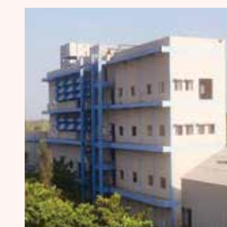
Multipurpose Plant No. 4 (exterior view)
