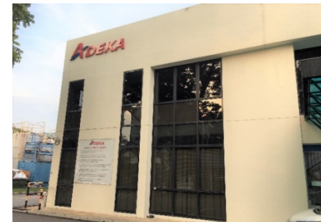
▲ The new processed food line in Singapore (exterior view of the production building)
