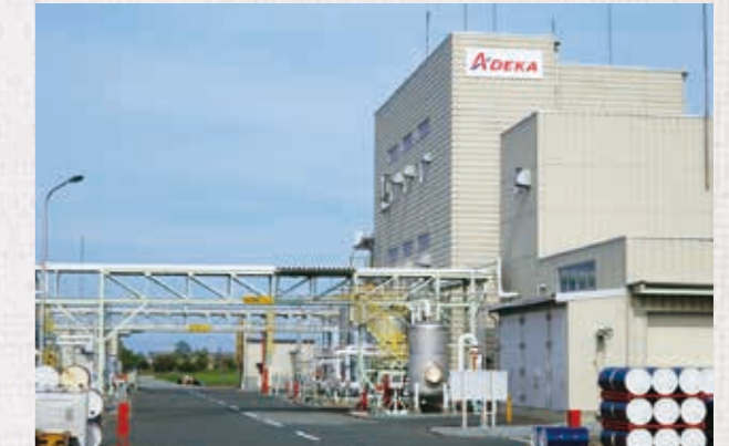
Soma Plant after reconstruction
