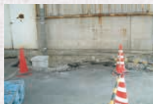
Kashima Plant suffering from ground subsidence as a result of the earthquake
