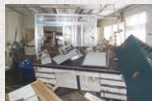
Soma Plant damaged by the tsunami
