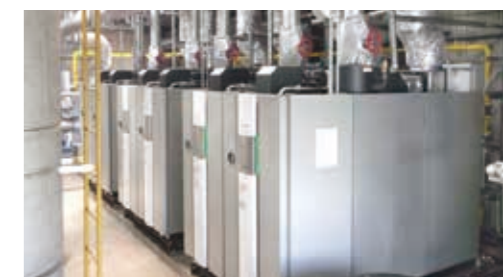
High-efficiency, energy-saving gas boiler facilities (Kashima Plant-West)
