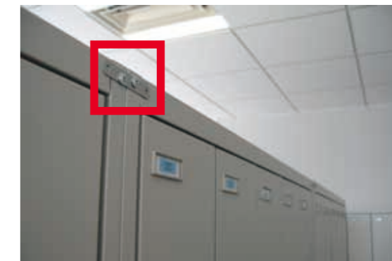
Measures to prevent employees' lockers from overturning
