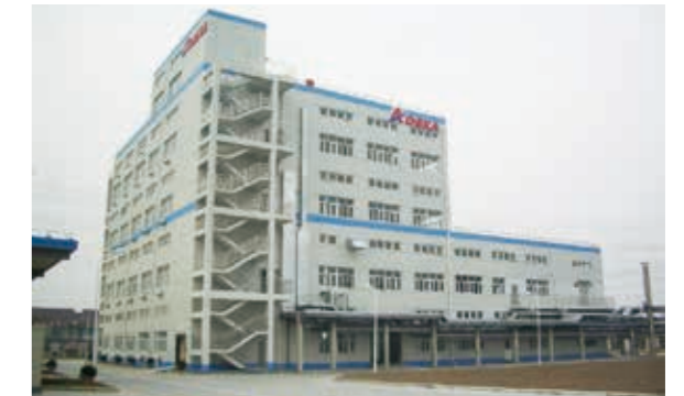
Production plant for flame retardants at Adeka Fine Chemical (Shanghai) Co., Ltd.
