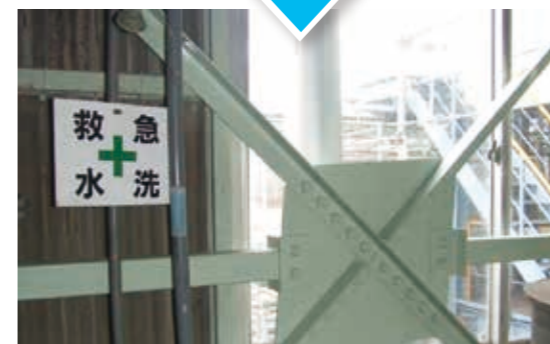
Seismic strengthening (Mie Plant)
