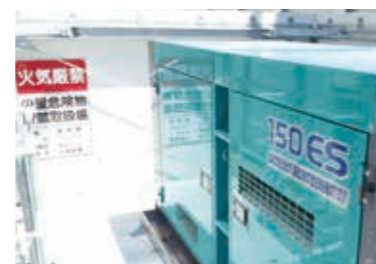
Introduction of privately-owned power-generating facilities (at the headquarters)
