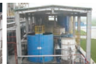
Phosphorus removal system at Adeka Fine Chemical (Changshu) Co., Ltd.
