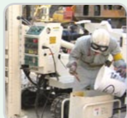
Soil and groundwater clean-up activities: Processing work involving microbial agent infusion
