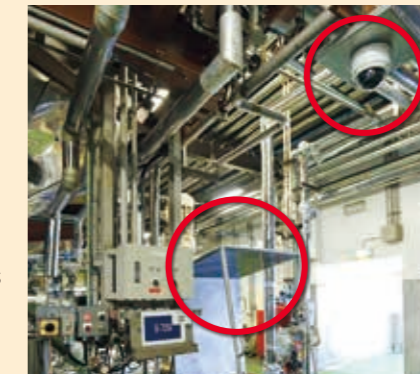
Installation of covers over the tops of raw material input ports, and setting up of monitoring cameras
