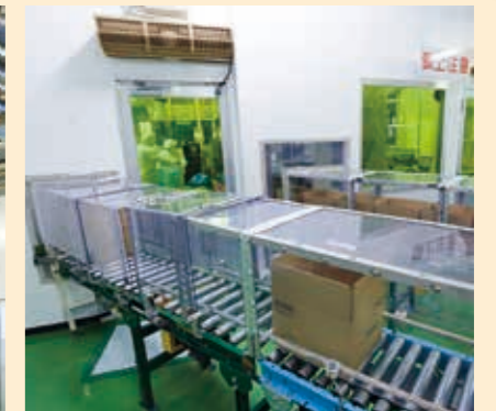
Installing tunnel-style covers over cardboard box conveyor lines
