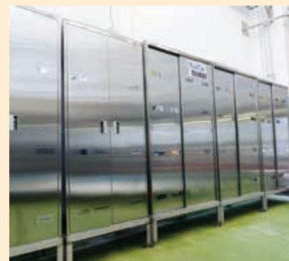
Securing spaces beneath the racks
